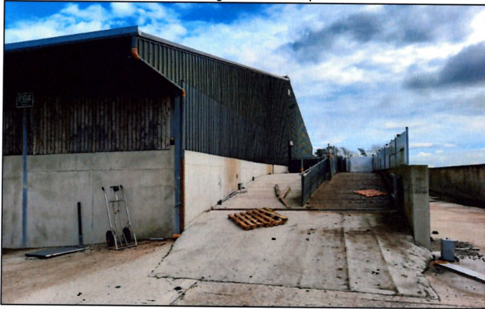
Existing shed with ramp
